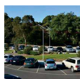
Square & Parking Solar Lighting
