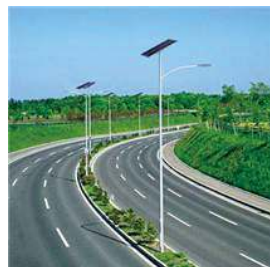
Solar Street Lighting
