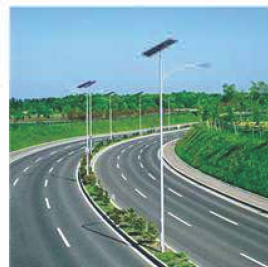
Solar Street Lighting
